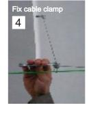
on jobsite, cut 1/16" (2mm) cable at a proper length, and fasten each end with a cable clamp.
