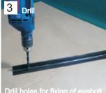
orill holes for fixing of nd expansion bolt
