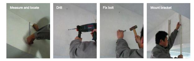
Determine the spacing and height of tension cable according to height and diameter of each metal duct outlet. Determination of bracket spacing requires that the front and the rear brackets of the same DurkeeSox system should be mounted parallel and symmetrically without any deflection.
