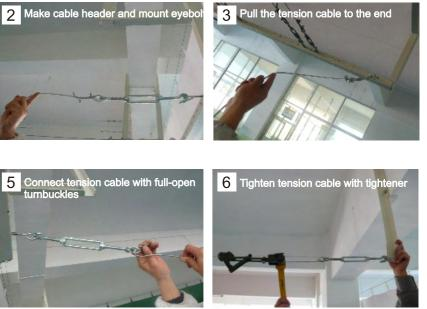
Note: Loose turnbuckle to the maximal when mounting cable suspension system to adjust the straightness of tension cable when under heavy load after installation of DurkeeSox system.
